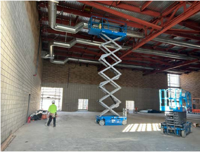
HVAC Ductwork Installation
