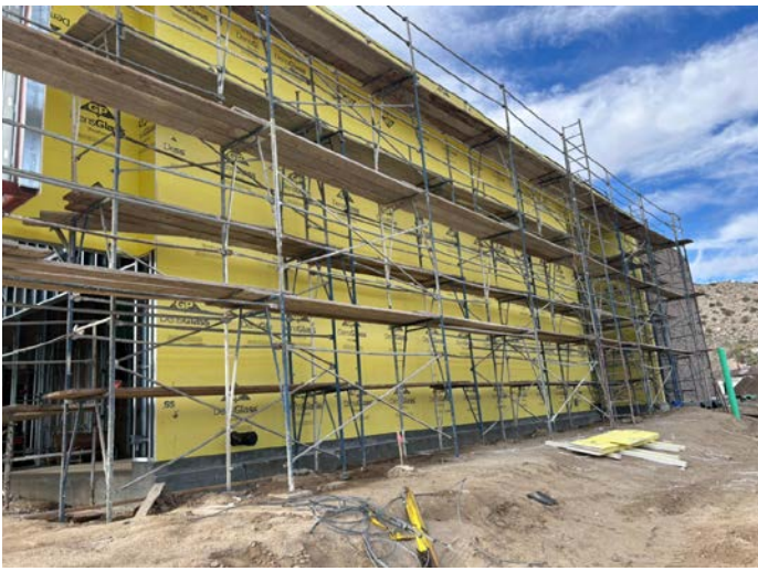
Segment 'A' Exterior Sheathing
