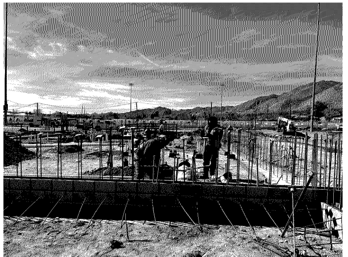
Concrete Masonry Starter Walls
