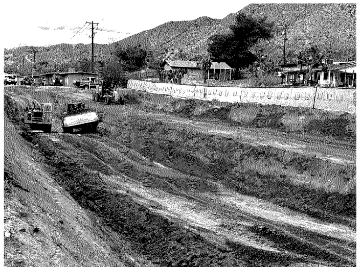
Over-Excavation at North West Side
