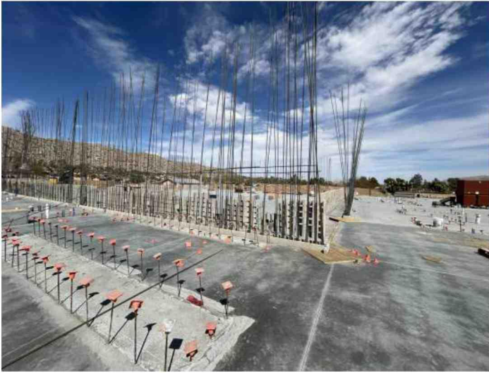
Start of Block Walls in Section A
