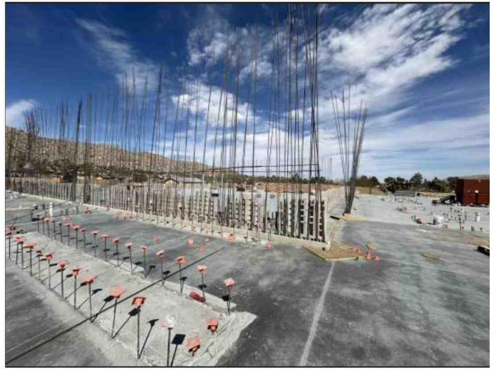
Start of Block Walls in Section A
