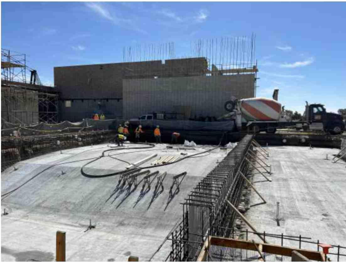
Block Walls for Sections A & C, Pool Walls Being Shotcrete
