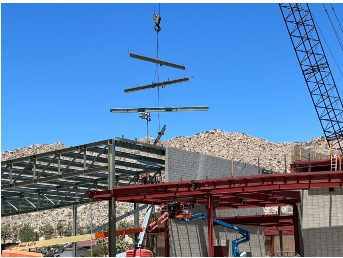
Roof Steel Erection Section B
