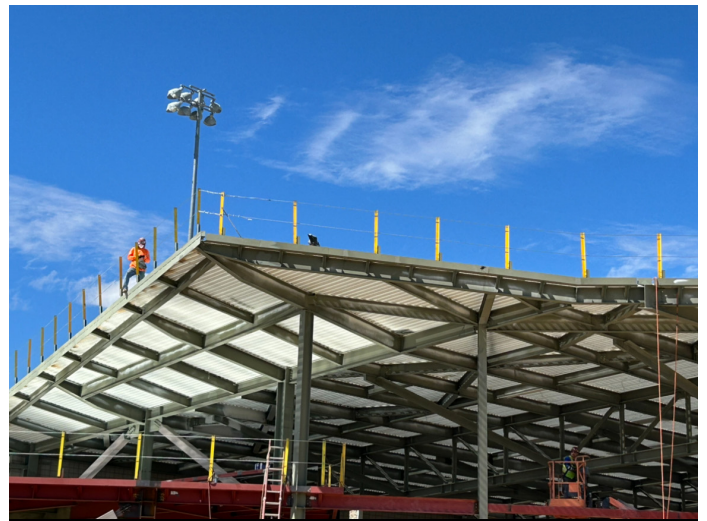
Segment 'B' Metal Decking Complete
