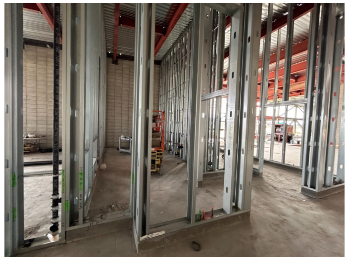
Section 'A' Interior Wall Framing
