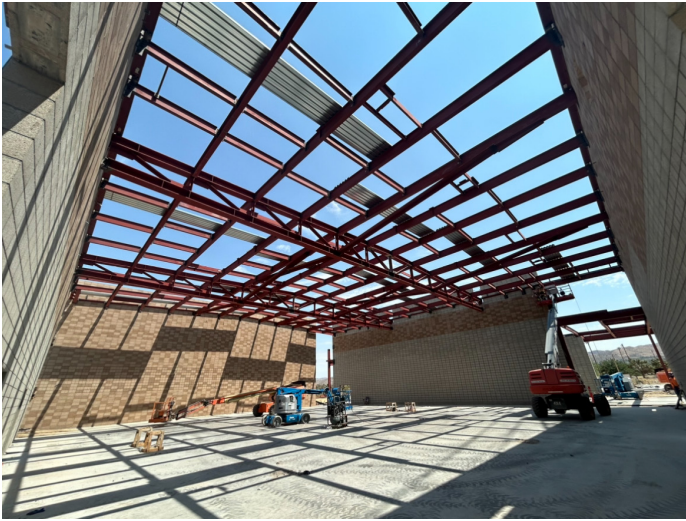
Segment 'A' Steel Roof
