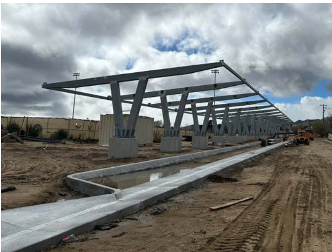
Solar Canopy Steel Erection
