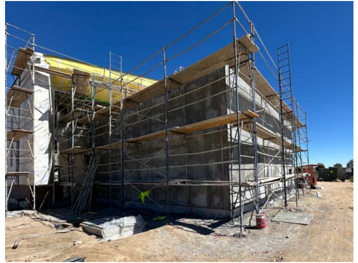
Segment 'B' Plaster Scratch Coat
