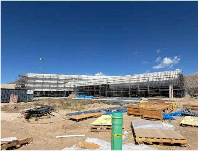
Building Weather Barrier
