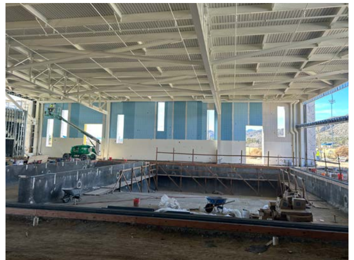
Natatorium West Wall First Coat of Paint
