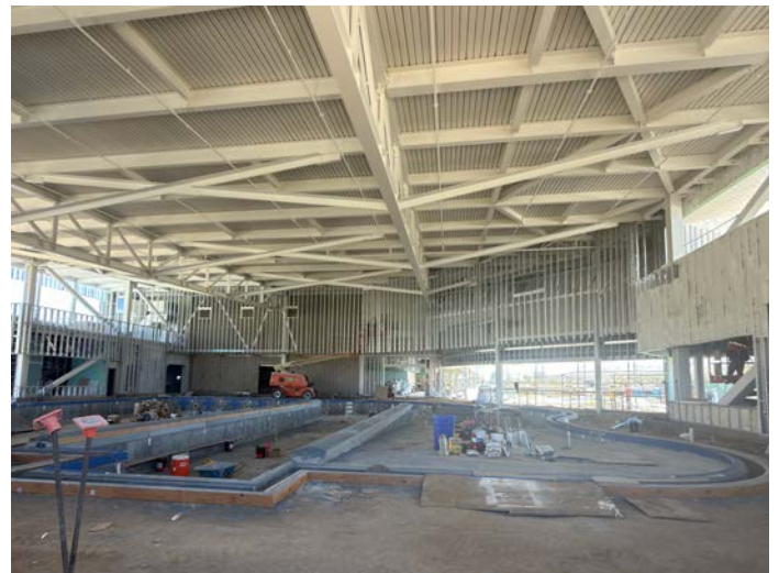
Natatorium Soffit and Pool Tile
